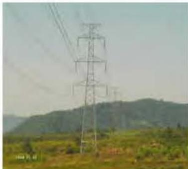
Fig. 4 Suspension Tower
