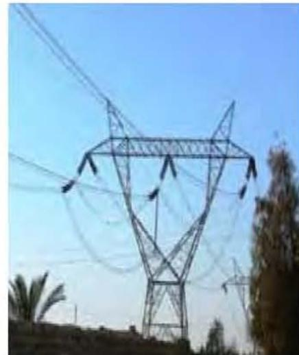
Fig. 5 Transposition Tower
